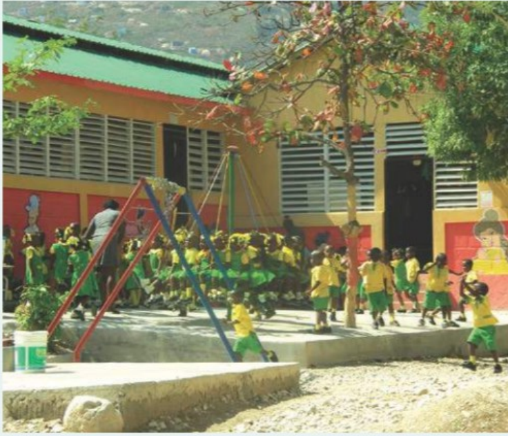
When the site could not accommodate three standardised school building blocks, on-site engineers were able to improvise effectively, designing a staggered arrangement without compromising safety. Photo: Bill Flinn.
